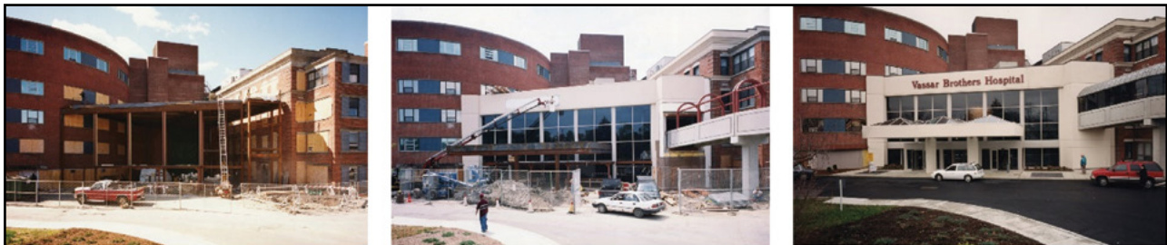
Main Lobby construction – April to December 1999 ©Berstein Associates, Photographers
