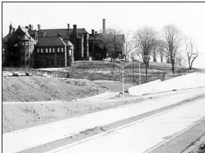
Construction of Route 9
